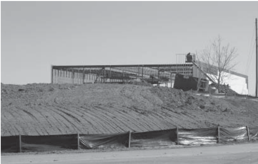
Commercial Construction, South Middleton Township
