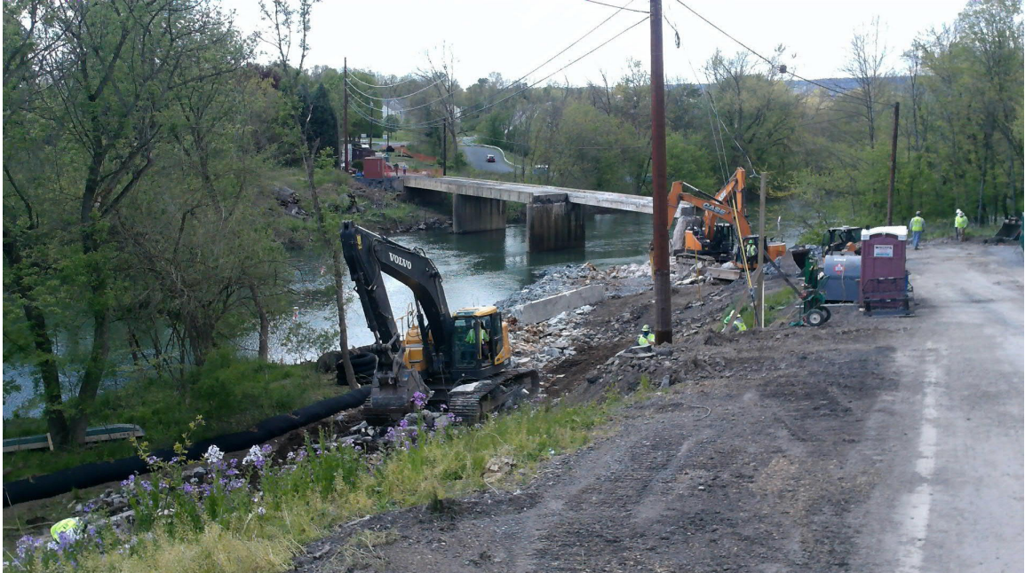
Span 4 Demo / Span 3 Partial Demo - Looking North -
