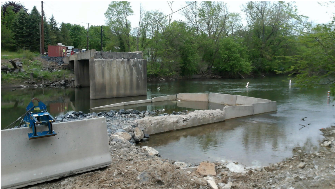
Cofferdam Installation – Pier 2 - Looking North -
