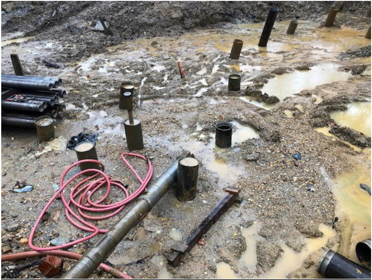
Micropile Installation
